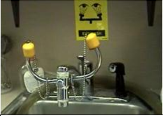
Readily accessible eye wash when working with corrosive chemicals
